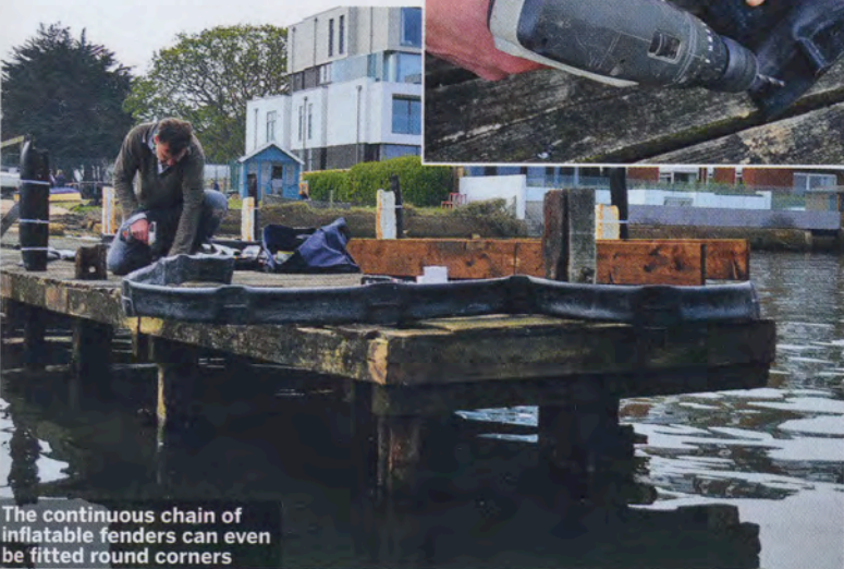
Once fixed in place, the fenders are easily inflated with a bicycle pump
